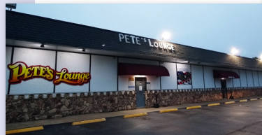
Ext. Building and Parking Lot Lighting
